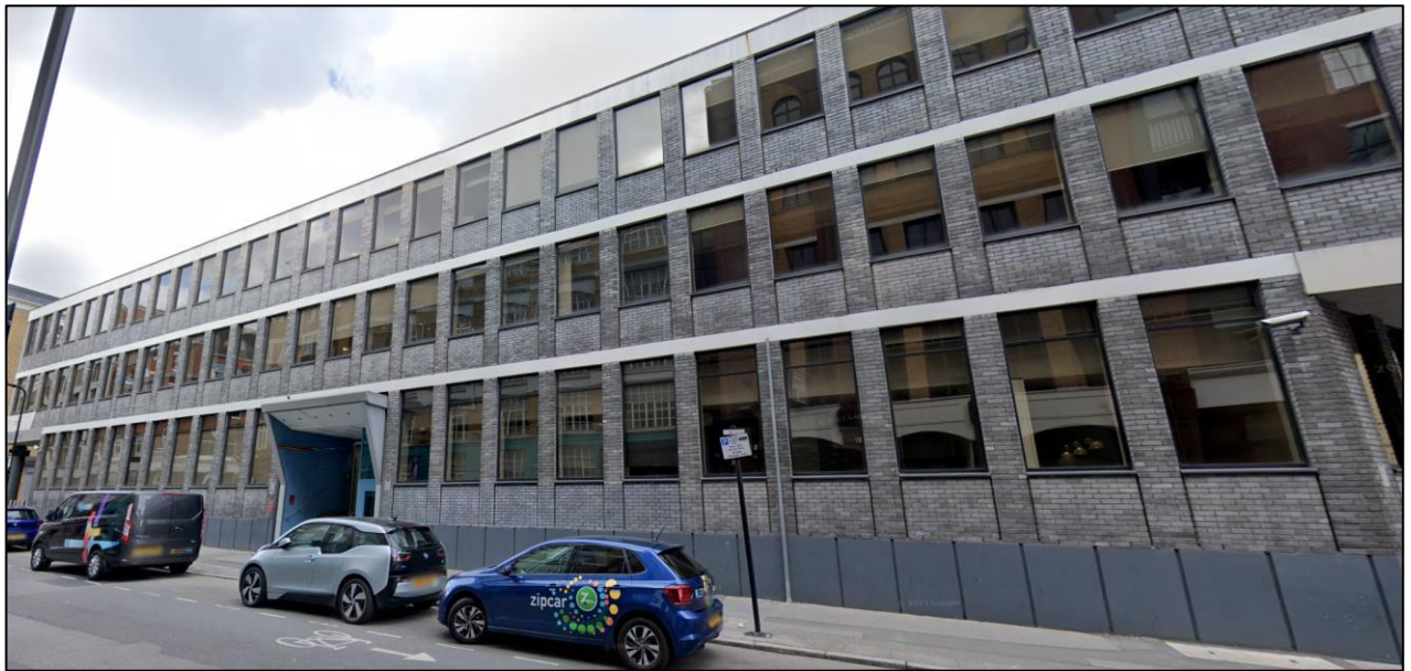
Figure 6: Paul Street elevation, looking south
