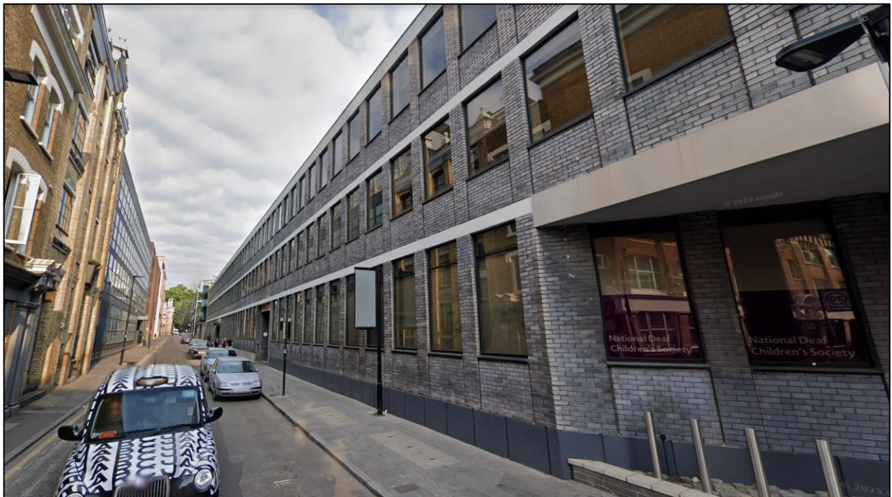
Figure 7: Epworth Street elevation, looking west
